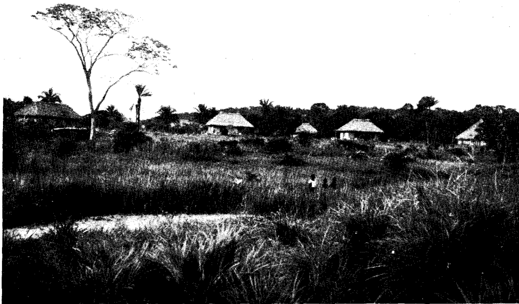
Brick dwellings at Inkongo. Left to right: Houses of Mr. and Mrs. H. Wilson, Miss Isaac, one for visitors, Mr. and Mrs. Downs. Other buildings hidden by trees. The long grass is used for thatching.
